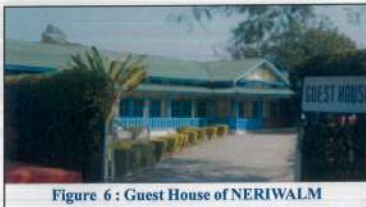
Figure 6 : Guest House of NERIWALM
