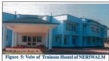
Figure 5: View of Trainees Hostel of NERIWALM
